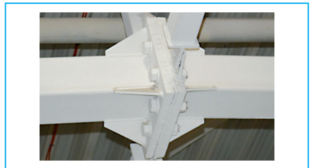
Steel structure treated with IK-6 intumescent coating
